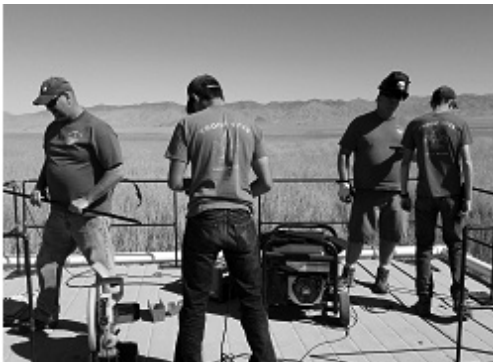
(l to r) Justin's father, Steve Cathey, Matthew Prince, Justin's Project Mentor and master welder, Ron Rockstrom, and Justin Cathey work on a black pipe frame that was constructed, welded to base plates and bolted to the deck of the dock.
